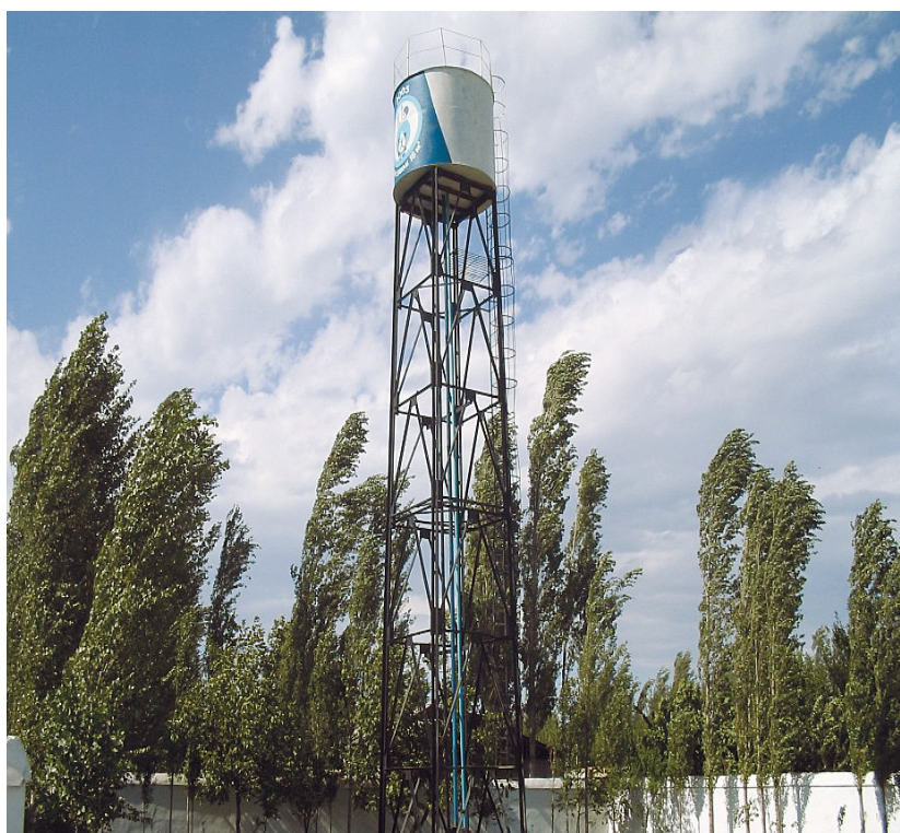
The infrastructure installed by the villages includes water reservoirs, such as the one in Kalainov.
