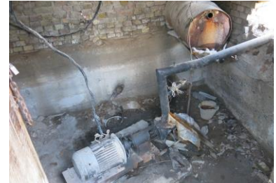
Inside of current pump-house and pump – to be rebuilt
