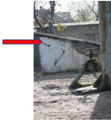
Old borehole pump-house – to be rebuilt
