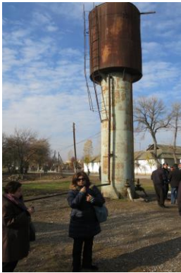
Old reservoir tower – to be rebuilt
