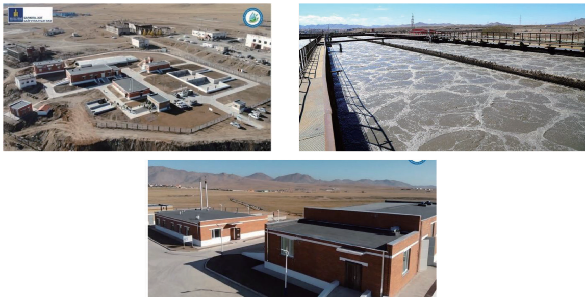
Figure 14. The new water supply and sanitation infrastructure for residents of Dalanzadgad Soum
