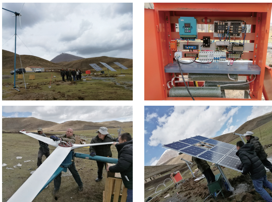
Figure 11. The Demonstration project in Gangchagongma Village
