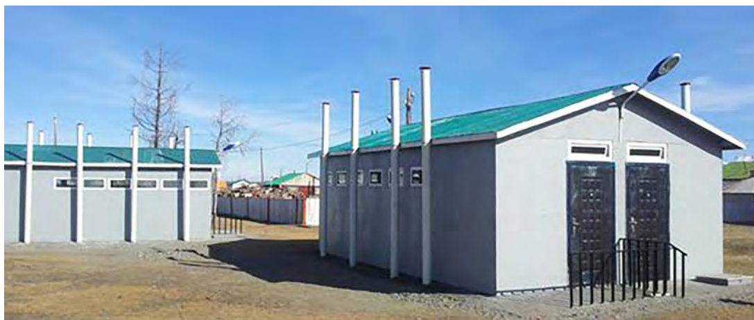
Sanitation blocks with dry toilets. The blocks are well insulated and ventilated with lighting (photo by Alcanz Consulting Group 2015).
