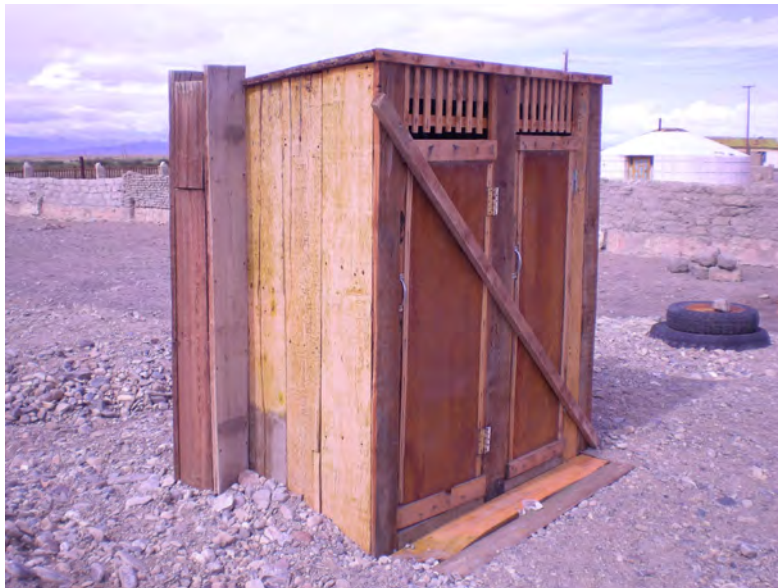
New pit latrine. Though the toilet is in better condition, there is still no place for children to wash their hands after defecating (photo by Kevin Tayler).
