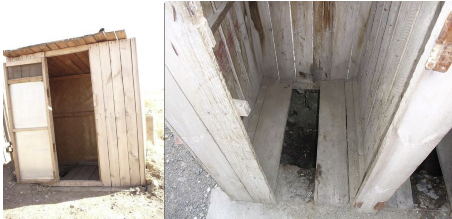
Fig. 4. Unimproved and unhygienic pit latrines in the Ger Areas (Field Survey, Uddin, April 2012).
