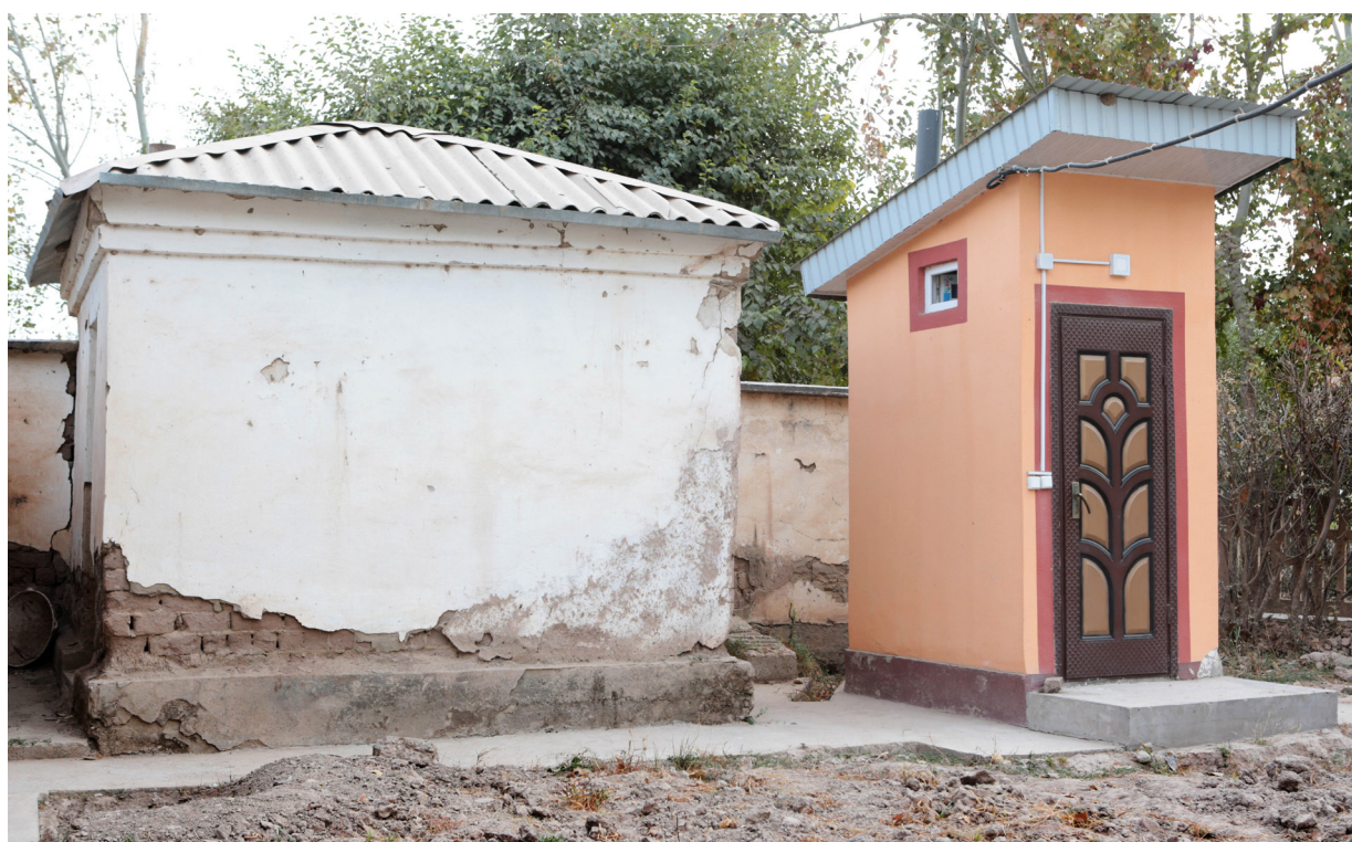
An upgraded latrine replacing an outdated facility. Photo credit: TajWSS
